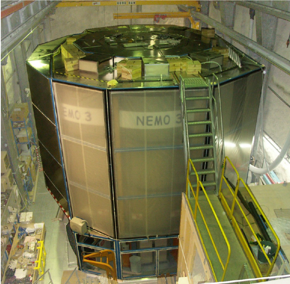
Figure 4.12: Picture of the airtight tent surrounding the NEMO 3 detector after its final installation in the LSM. As shown in this picture, the lower part of the tent which surrounded the electronics is now removed.
