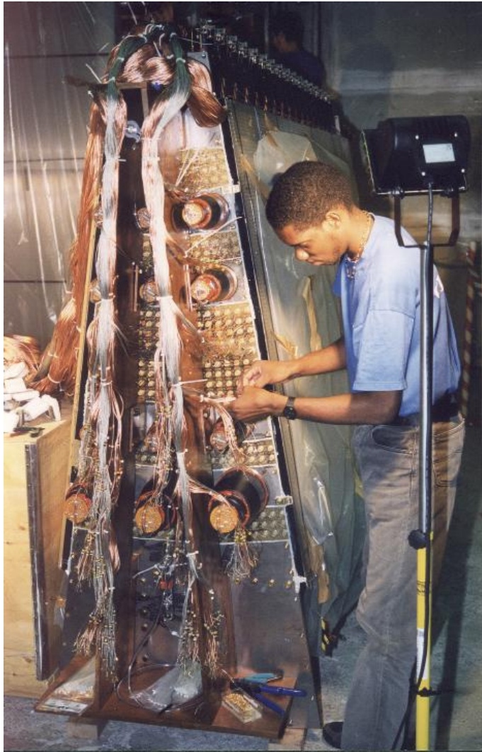
Figure 2.37: Picture of the anode and cathode cabling in LAL.
